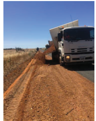
Works Construction Crew
