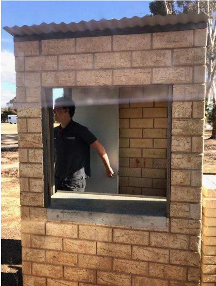
It was agreed that a permanent ticket box structure was required on the southern entrance of the main Spoetsground entrance. The structure to be built in brick with a colorbond roof. The building to provide a place to sell tickets from both the pedestrian side gate and the vehicle entrance. The structure will also provide shelter over the pedestrian access.
